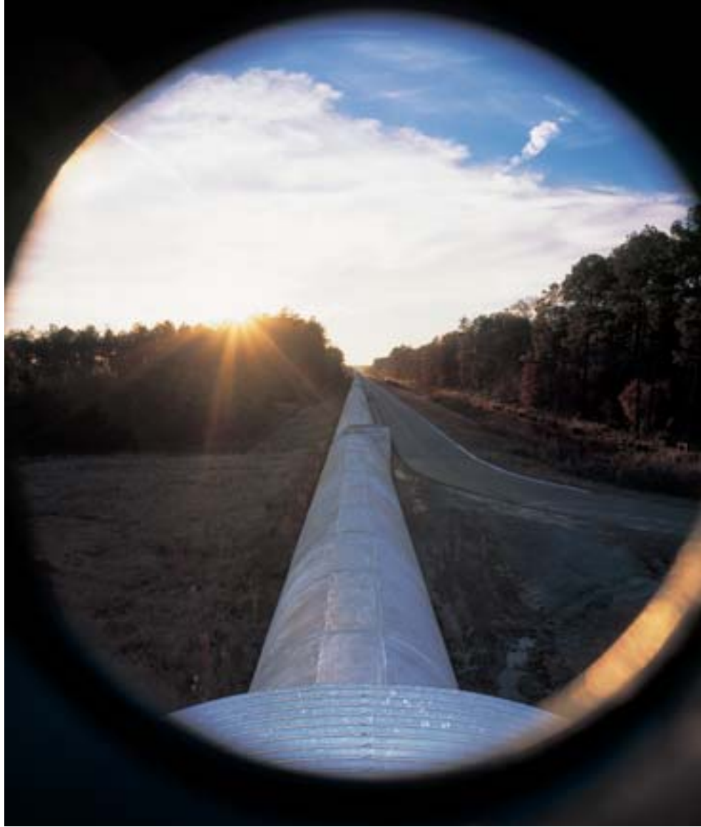
STRAIGHTER THAN THE SURFACE OF THE EARTH , the concrete tunnel that houses the west arm of the LIGO Livingston Observatory rises more than a meter off the ground on its four-kilometer run as the planet curves beneath it. The tunnel houses an airtight steel pipe. Inside the pipe is a vacuum, and through the vacuum shines a beam of infrared light with the power of 20 million laser pointers.
